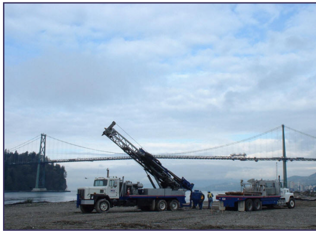
Truck Mounted AP-1000 H180 Becker Hammer Rig
